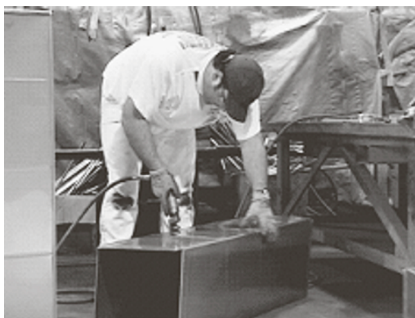
Figure 1-1.10. Using the floor as a workbench
