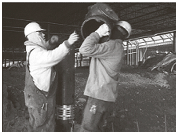
Figure 1-1.9. Carrying or lifting heavy materials
