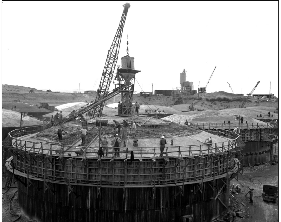
Figure 1: Waste Storage Tanks under Construction at DOE's Hanford Site, September 1947
