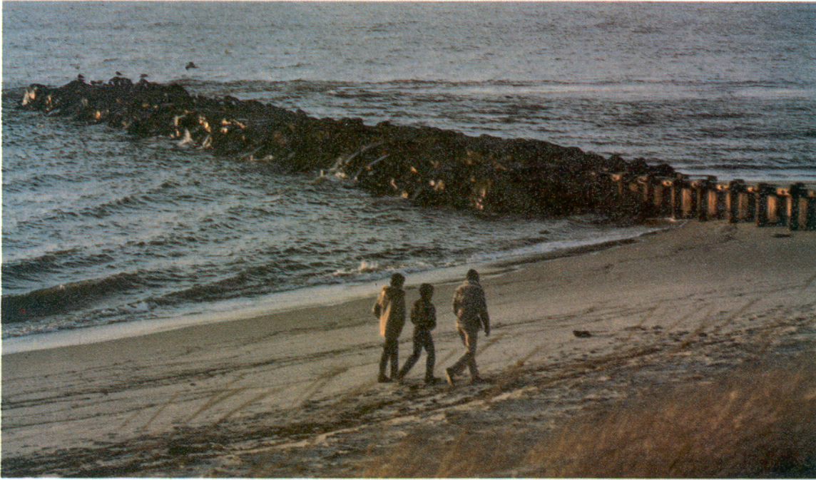
Treated-timber and rubble groin
