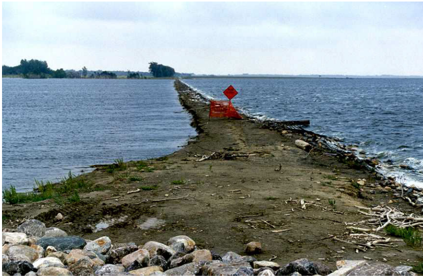
Stromme's Road, Looking East From Highway 20/57
