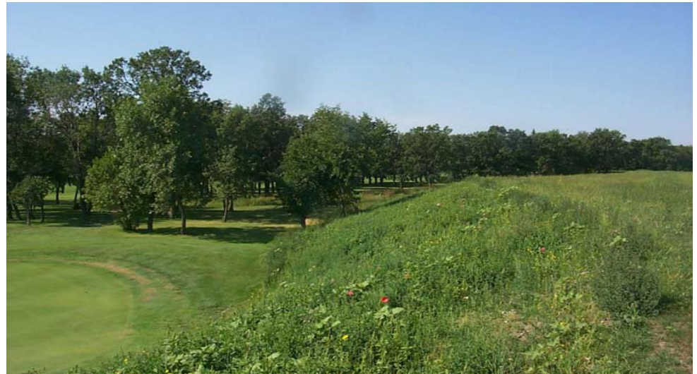
Embankment at Golf Course
