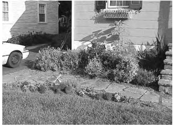
Recently planted raingarden treating residential rooftop runoff
