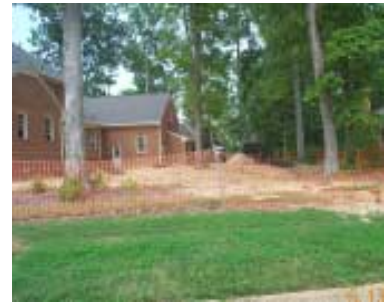
Limited site clearing in VA.
