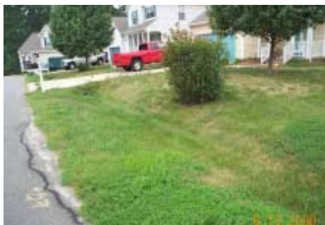
Vegetated open channel in Springhill, VA.
