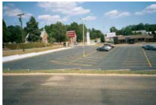
Example of excess parking construction.
