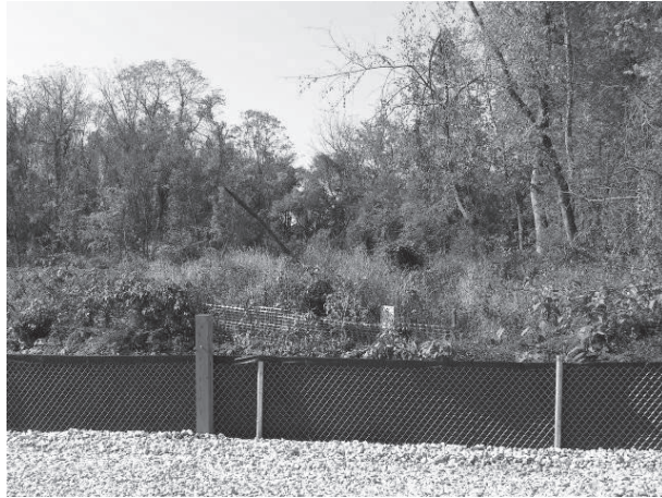
Properly installed erosion control fences are critical to protecting waterways and natural areas from sediment pollution.
