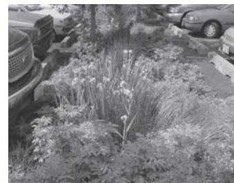
A parking lot bioretention area infiltrates and reduces stormwater runoff pollutants.
