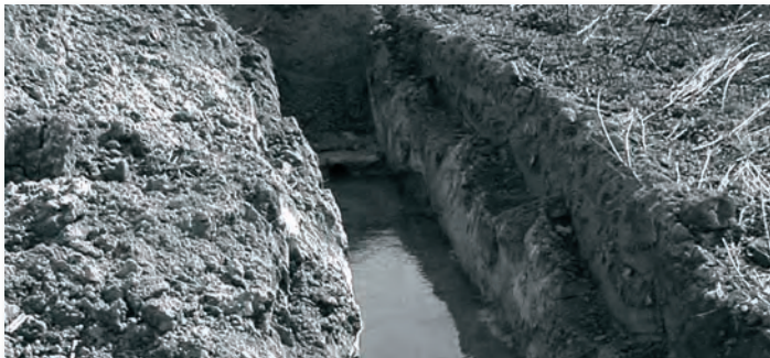
Photo showing trench where drain tiles have recently been excavated. It is important to fill this area back in with soil to avoid a drainage conduit.
