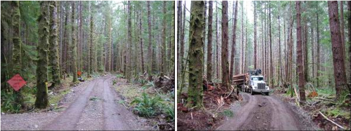
Figure 8. Pictures of temporary roads during use.
