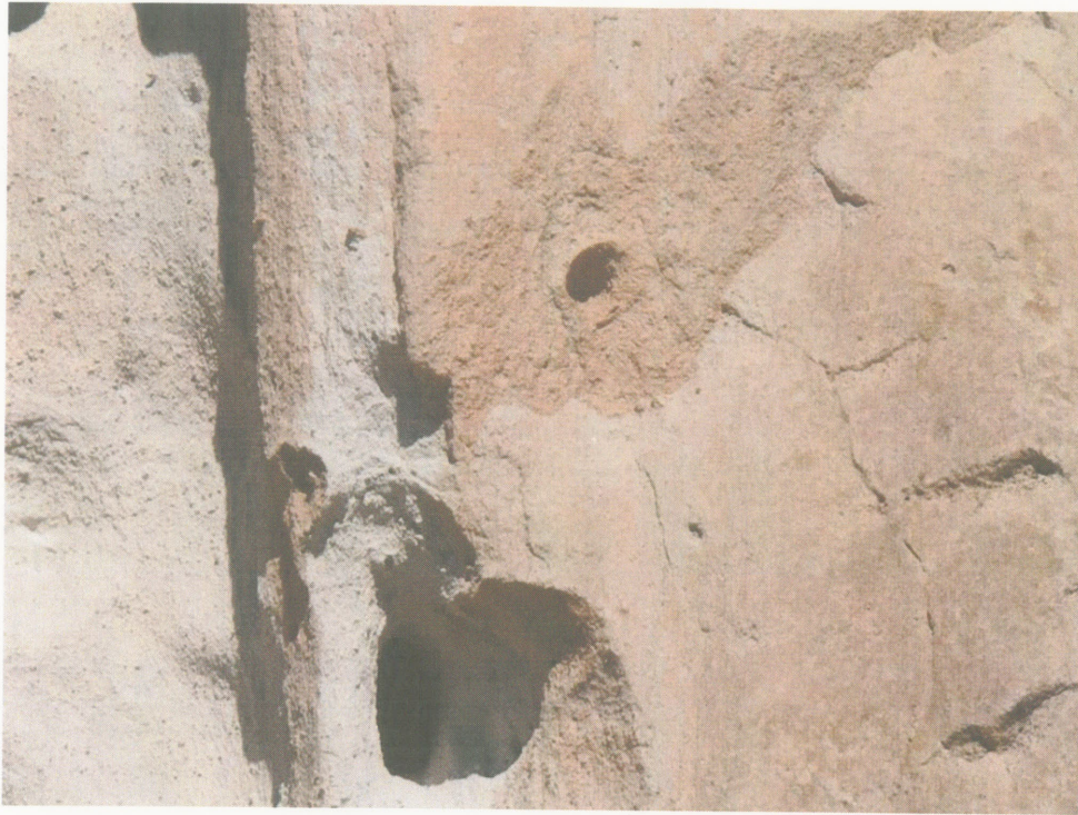
SWMU-011(e) cliff face target area.
