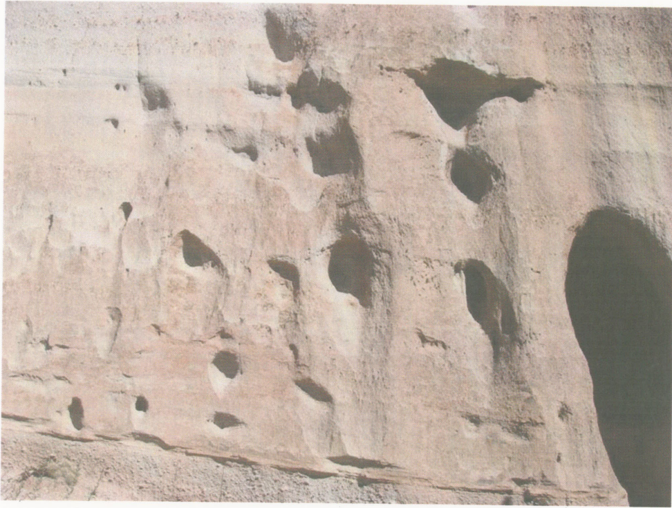
SWMU-011(e) cliff face target area.
