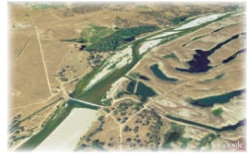
Antiquated fish ladders at Daguerre Pt. Dam impede fish passage.
