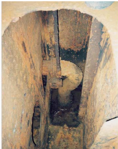
Photo 2.2: Deep transverse floors vertically stiffened in after peak tank. Note ballast line leading to bellmouth.
