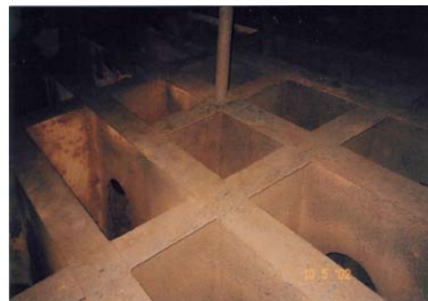
Photo 2.29 and 2.30: Deep floors and girders within a forepeak tank providing additional strength to the forefoot are particularly conducive to mud accumulations but more readily accessible for washing down.
