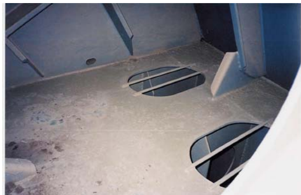
Photo 2.28: Side tank stringer plate. The absence of drainage around the perimeter, and particularly along the connection to the shell plating results in sediment accumulation over a relatively large area of plating.
