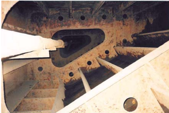
Photo 2.4: Transverse and longitudinal framing within a topside tank.
