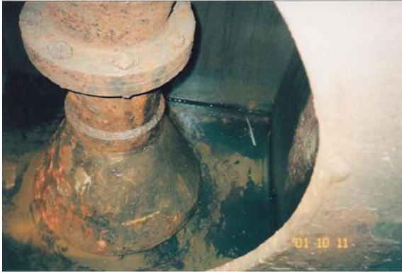
Photo 2.6: Typical bellmouth installation in a forepeak tank. See also Photo 2.2.
