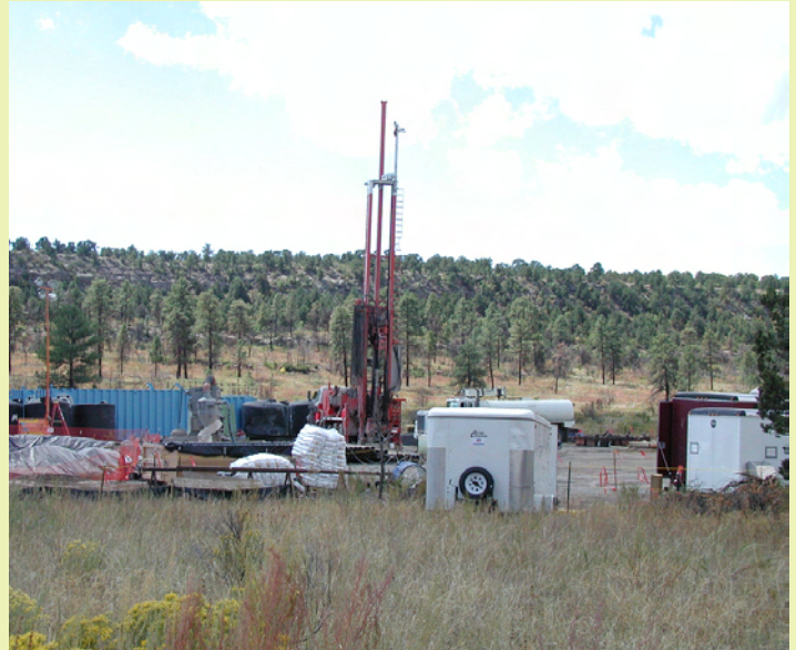
Drilling a well in Mortandad Canyon
