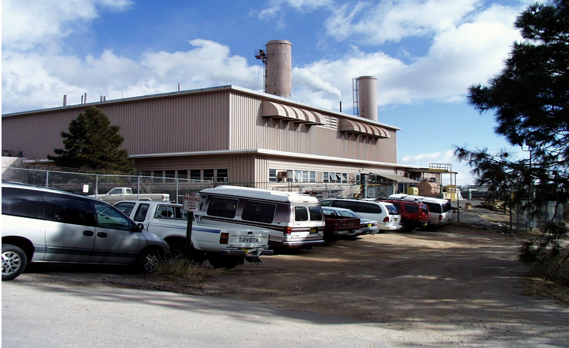
Figure 2-1. Main steam plant at LANL TA-3.
