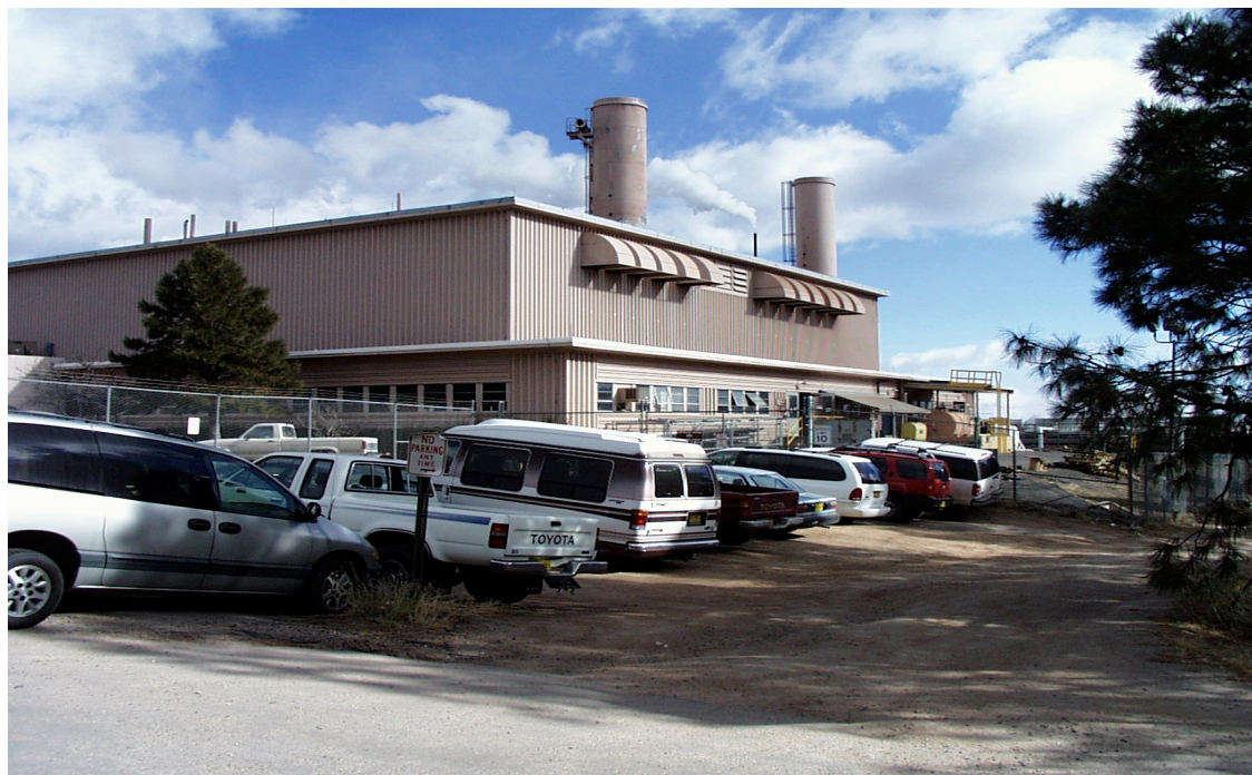
Figure 2-1. Main steam plant at LANL TA-3.
