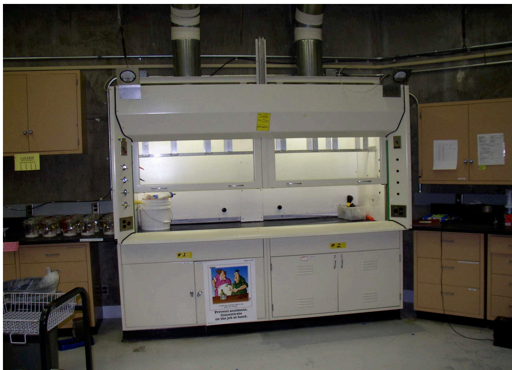
Figure 2-2. Example of chemical use in laboratory hood at LANL.
