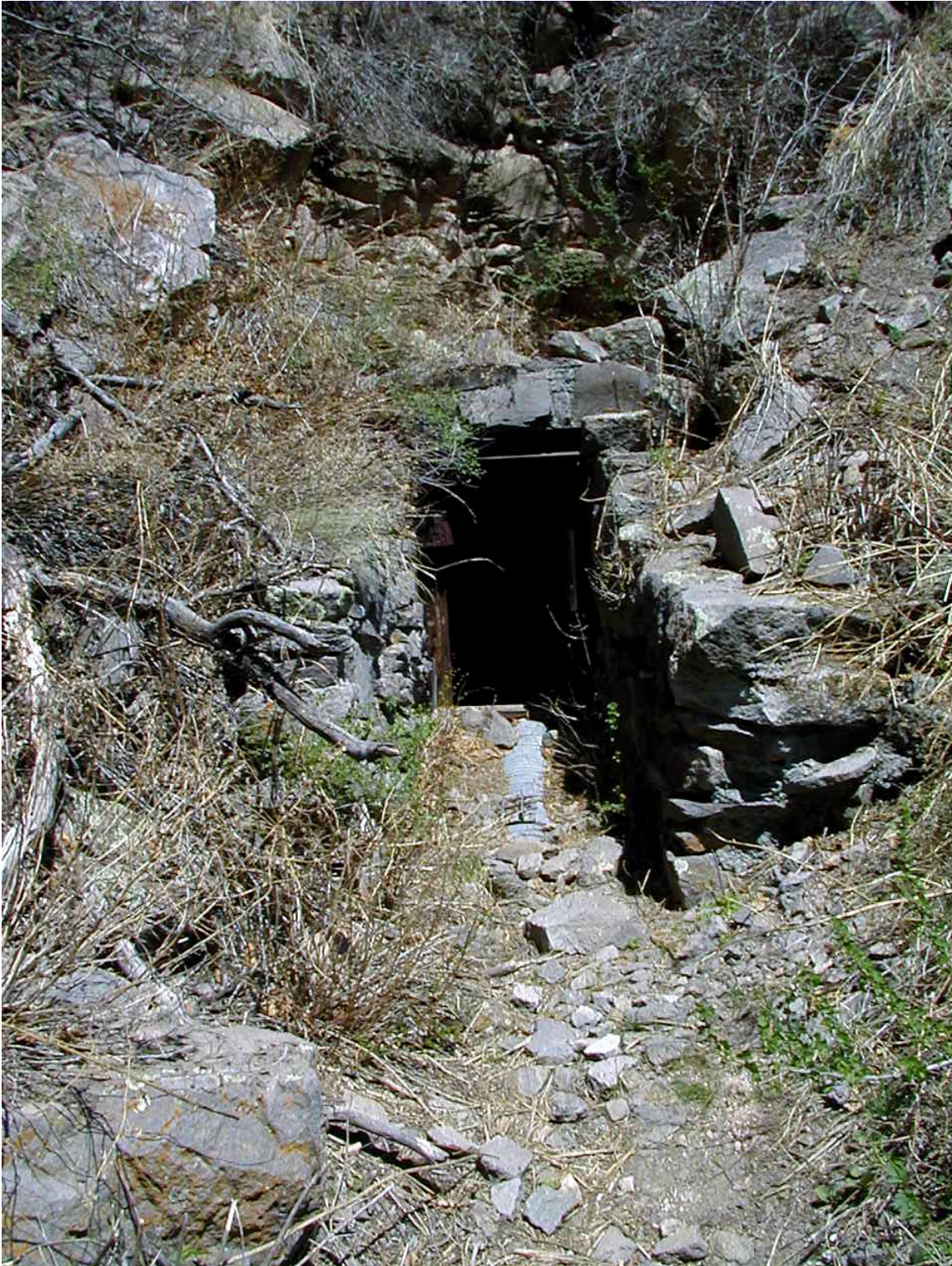
Figure E-6.1 Photograph of the entrance to Water Canyon Gallery taken on April 27, 2000.
