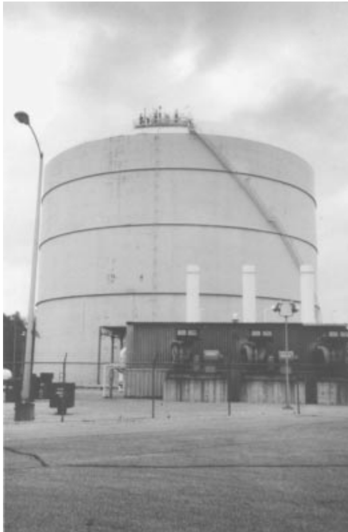
Liquefied natural gas (LNG) is stored in production facilities.
