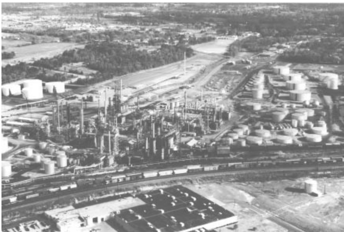
An overhead view of a natural gas processing plant.
