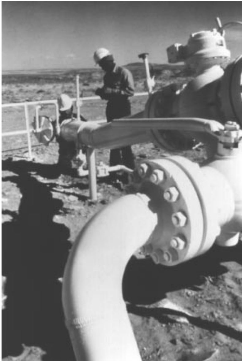
Workmen adjust valves on a Panhandle Eastern pipeline.
