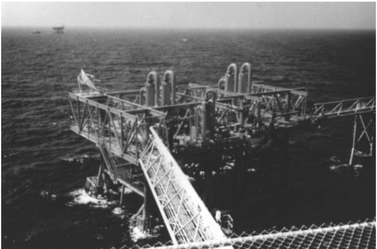
This offshore natural gas production platform is located in offshore Louisiana.
