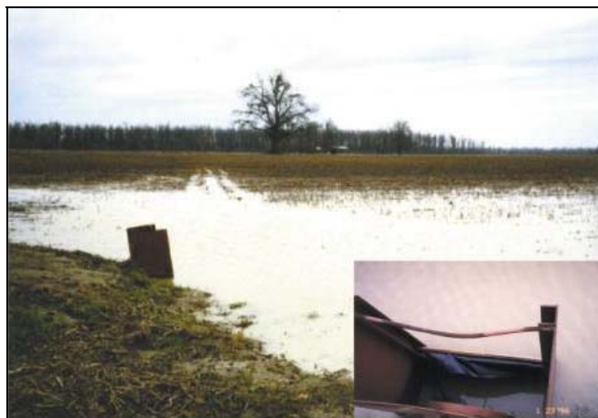
Figure 5. A slotted-board riser is a box welded to the inlet of a pipe that controls the surface runoff where it leaves a cropped field. Boards inserted into the control box hold water in the field during the winter, creating waterfowl habitat and allowing sediment to settle.
