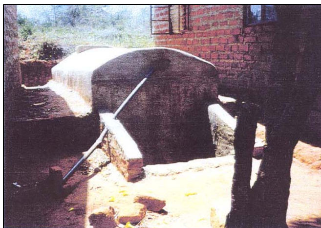
Figure 5: Roof harvesting into sausage tank - Machakos District.
