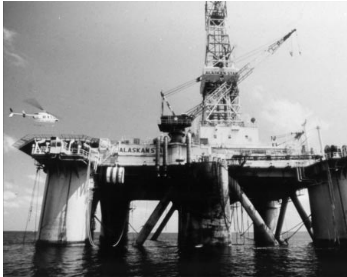
Semisubmersible drilling rig in the Gulf of Mexico. Source: U.S. Department of Energy.
