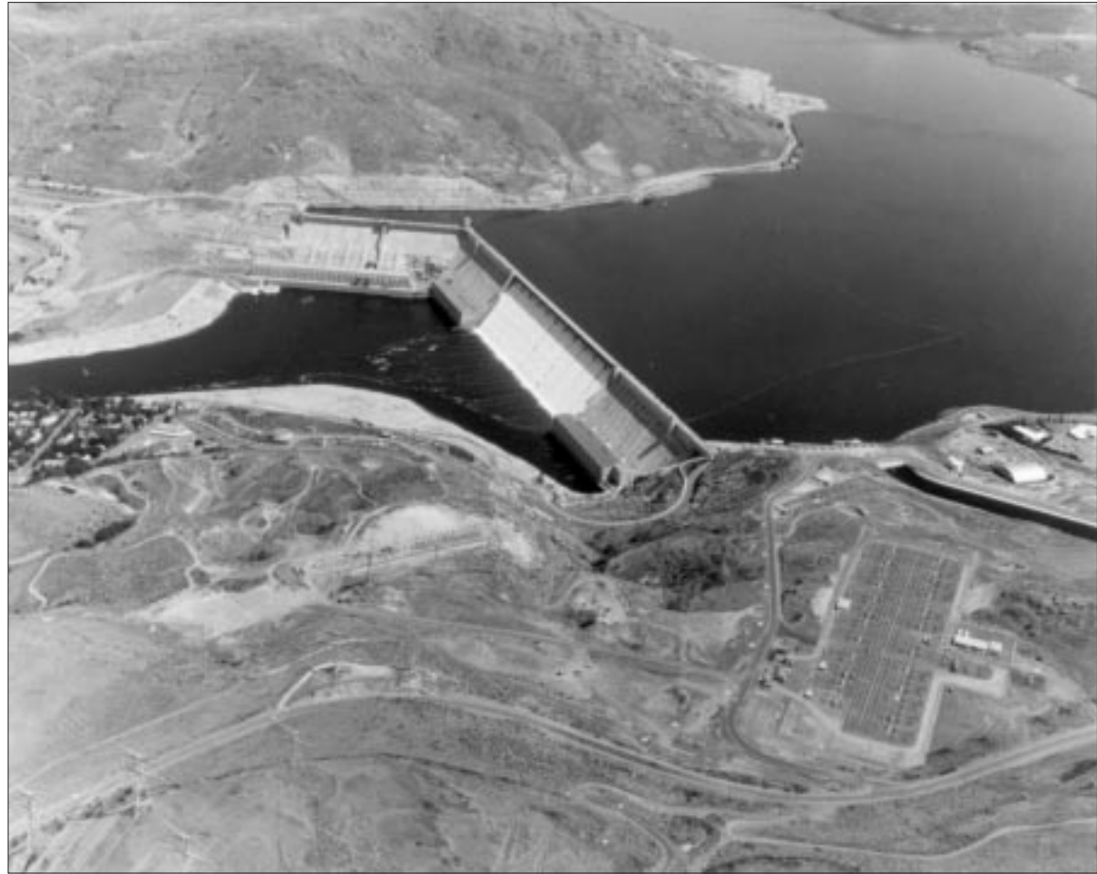
Grand Coulee Dam, Washington State. Source: U.S. Bureau of Reclamation.
