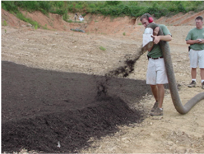
Examples of compost filter berms.
