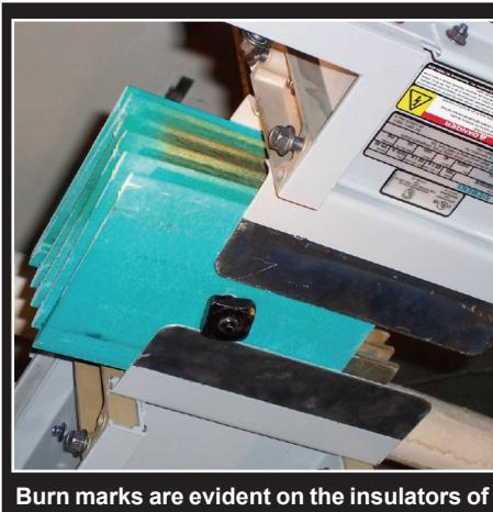
Burn marks are evident on the insulators of the 480 volt electrical buss at HRL.
