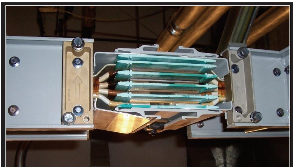
Incorrectly configured joint on buss raceway
