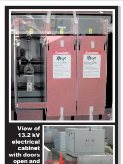
explosion and plasma fireball that would have been directed outside the cabinet doors and likely have incinerated anything within 15 feet of the open door.
