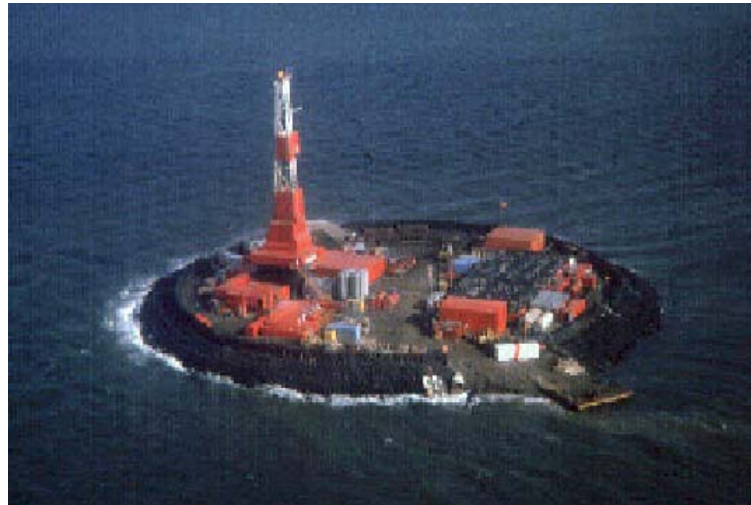
Land drilling rig on a man-made gravel island, Beaufort Sea, Alaska
