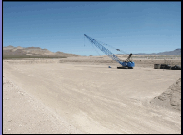
Pit 16 at the Area 5 Radioactive Waste Management Complex.
