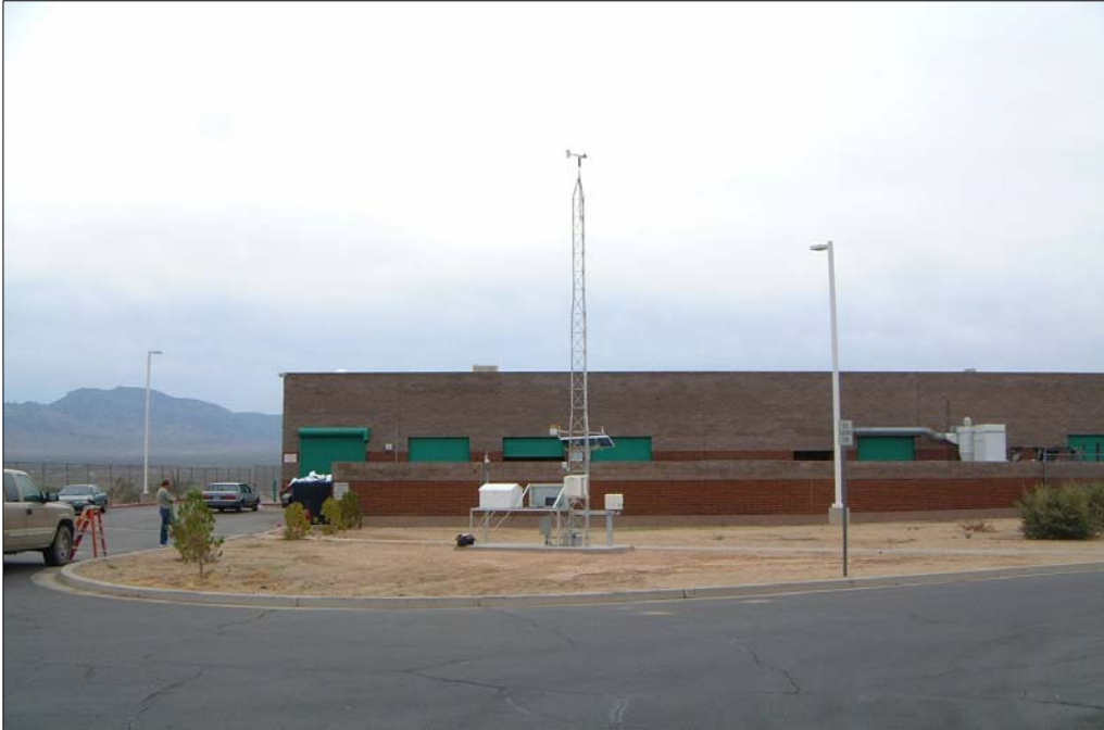
Figure 6-2. CEMP station at Mesquite, Nevada
