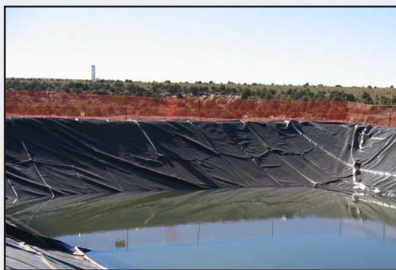
Lined Tritium-Contaminated Groundwater Containment Sump at an Area 20 UGTA well (photo by Russell Shelton, November 2005)
