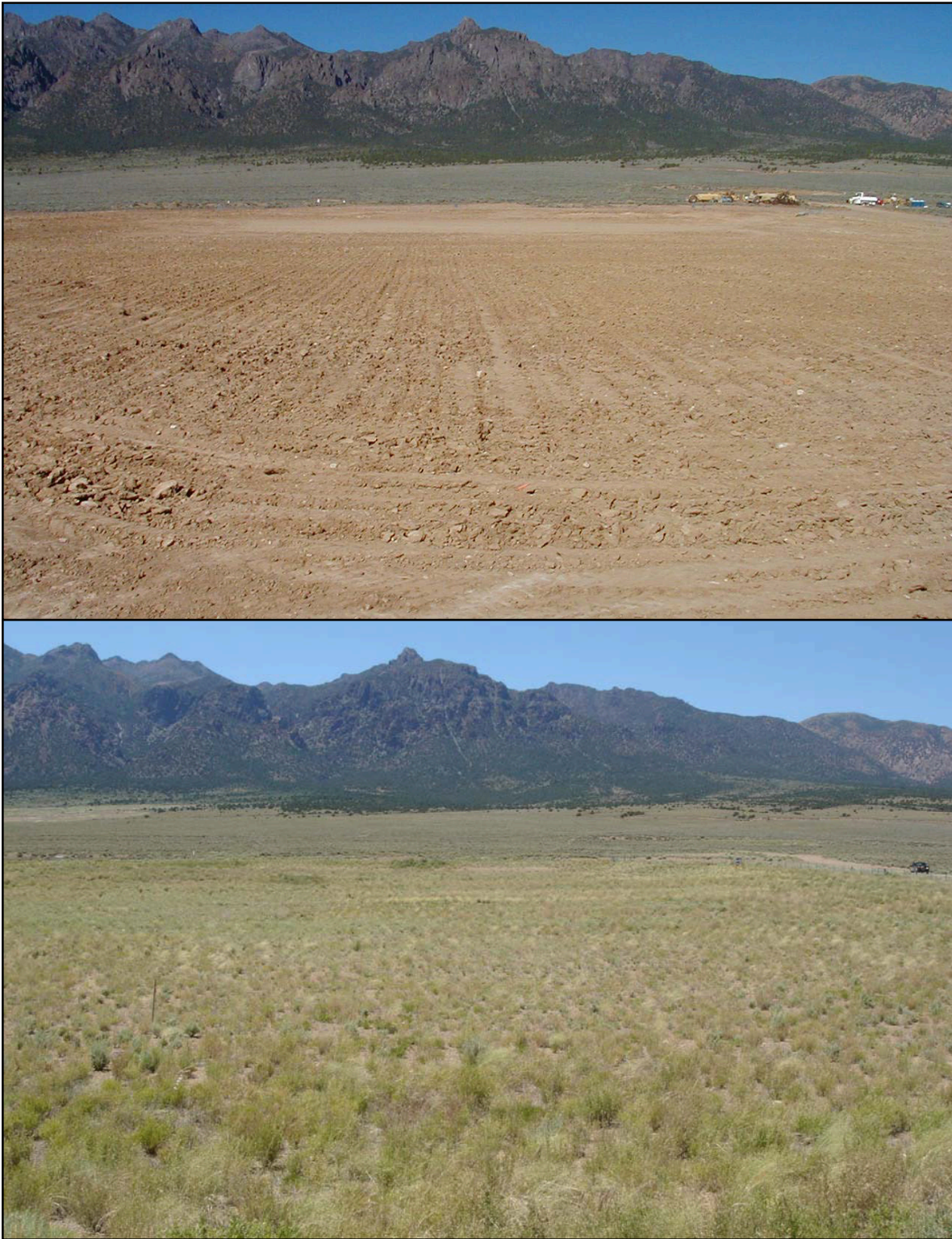
Figure 8-2. CANTA closure cover cap in 2000 following site preparation and seeding (top photograph) and June 2006 (bottom photograph). (Photographs by D. C. Anderson, October 2000 and June 2006)
