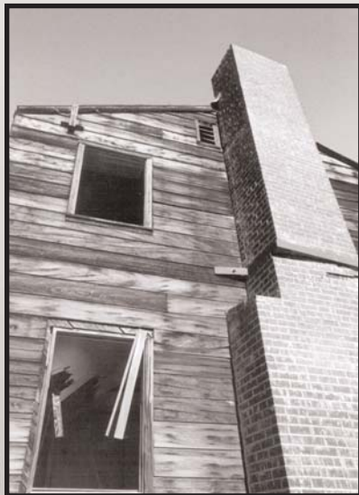
The remains of this Apple 2 two-story wooden house may be viewed on a public tour of the Nevada Test Site.
