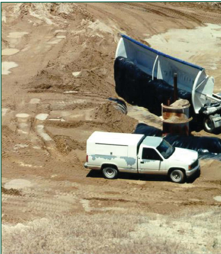
Clean Slate I soils shipment packaged in a soft-sided bulk waste container and disposed at the Area 3 Radioactive Waste Management Site.
