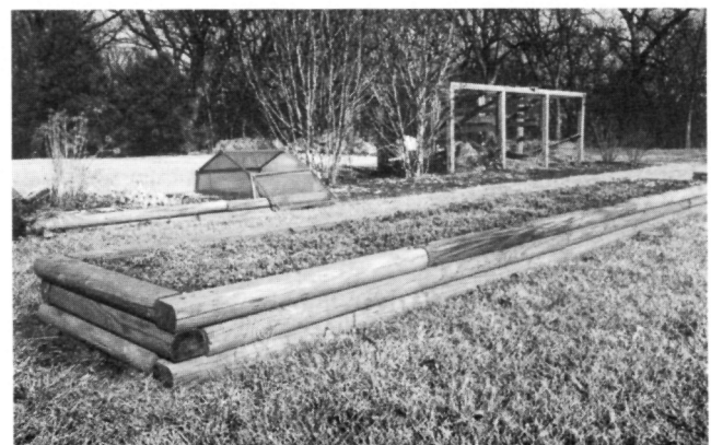
B. Reinforcing Rods Hold Timbers Together.
