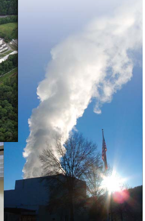
After more than a year of being shut down, the plume from the HFIR cooling towers—indicating operation—was a welcome sight.
