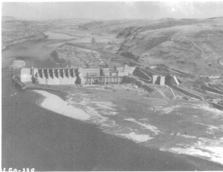
LITTLE GOOSE LOCK AND DAM DURING CONSTRUCTION 1968
