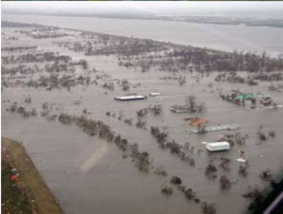
Flooding damage due to Hurricane Katrina.
