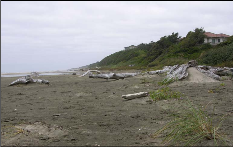
A New Shoreline Structure GIS Database developed by the Oregon Coastal Management Program will assist local planners and state agency staff with long-range planning on Oregon's beaches.
