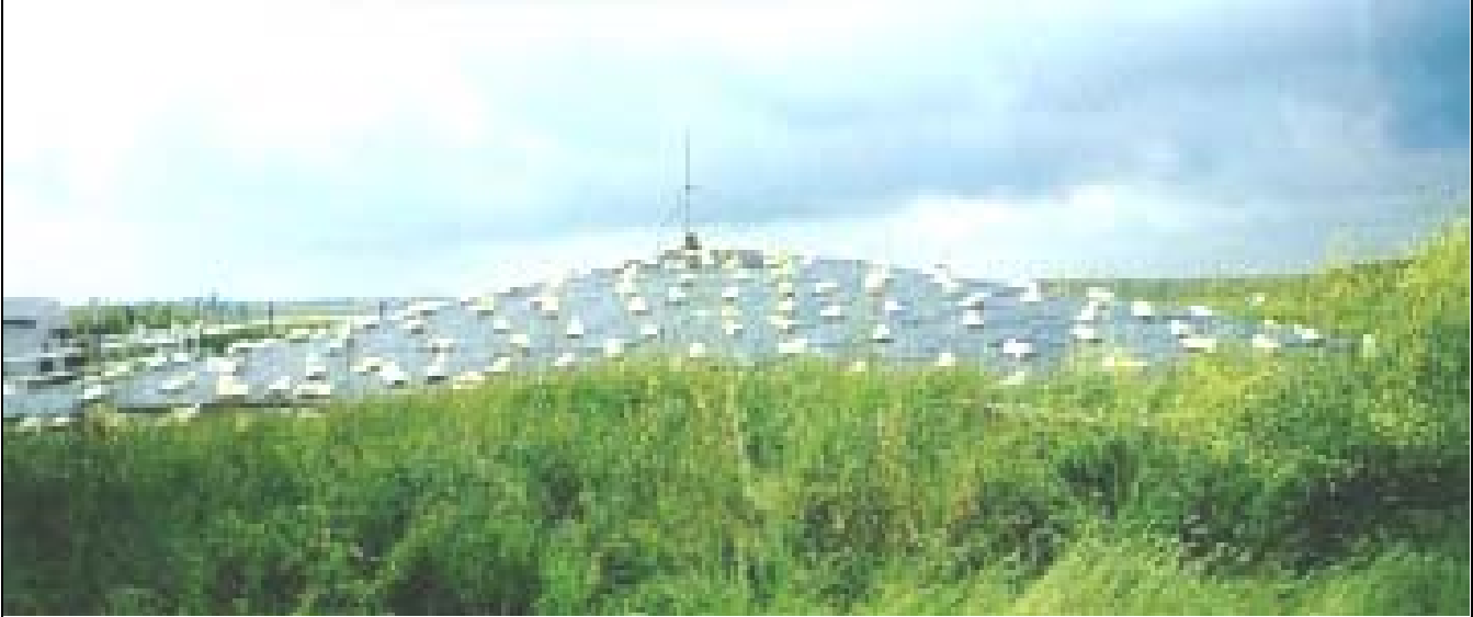
Landfill bioreactor cell, Yolo County, California
