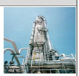
Nitric-acid plant controls for  $NO_x$  using both nonselective catalytic reduction and selective catalytic reduction technologies. Nonselective catalytic reduction is very effective at controlling  $N_2O$ .
