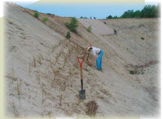
Several different seeding methods were tested on the slope
