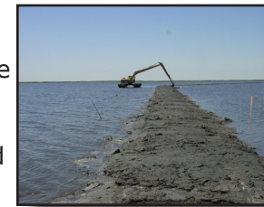
Construction of earthen terraces on CS-32 project
