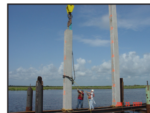
Concrete wall on BA-27 Project
