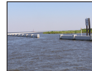
Completed concrete wall on BA-27c project
