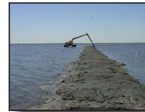
Construction of earthen terraces on CS-32 project
