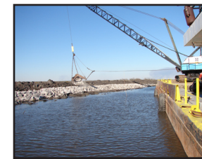
Construction of rock dike on the TE-46 project
