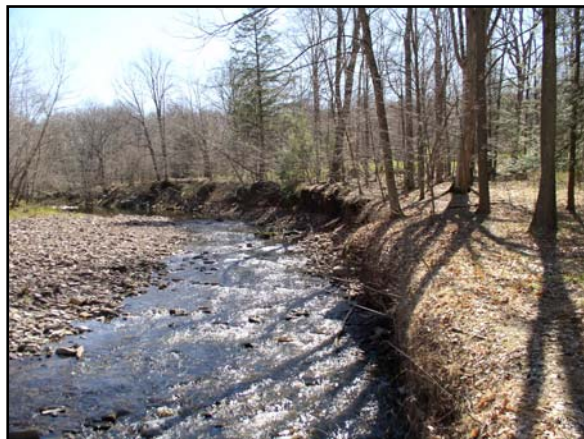
Streambank Erosion on Lower Wickechoke Creek
