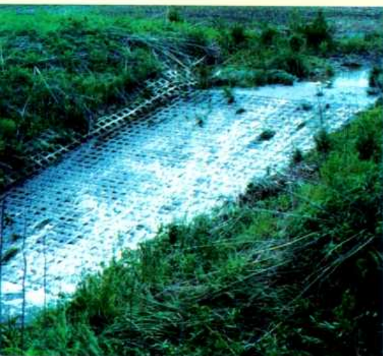
Concrete blocks can be placed by the owner to form a chute structure. This can be an inexpensive option to help stabilize an eroding gully.
