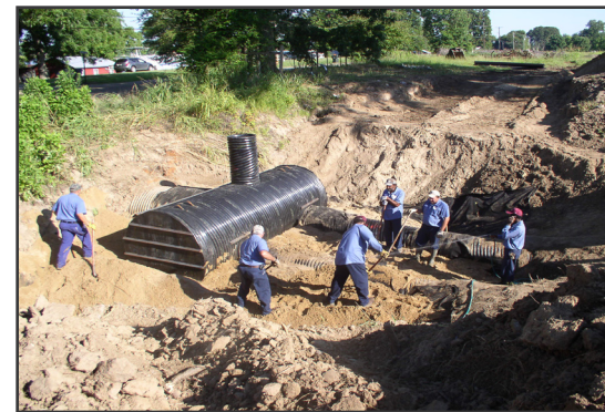
Installation of an erosion control structure along LA-413
