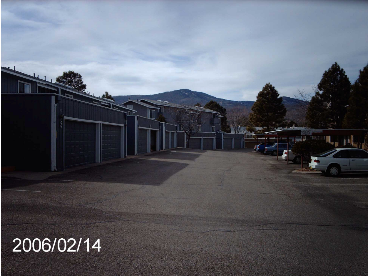
Figure 4.3-2. SWMU 01-001(b) mesa top site photograph (looking west)
