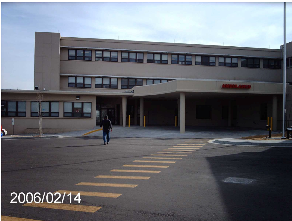
b) Looking south, line 171 runs beneath parking north of LAMC
