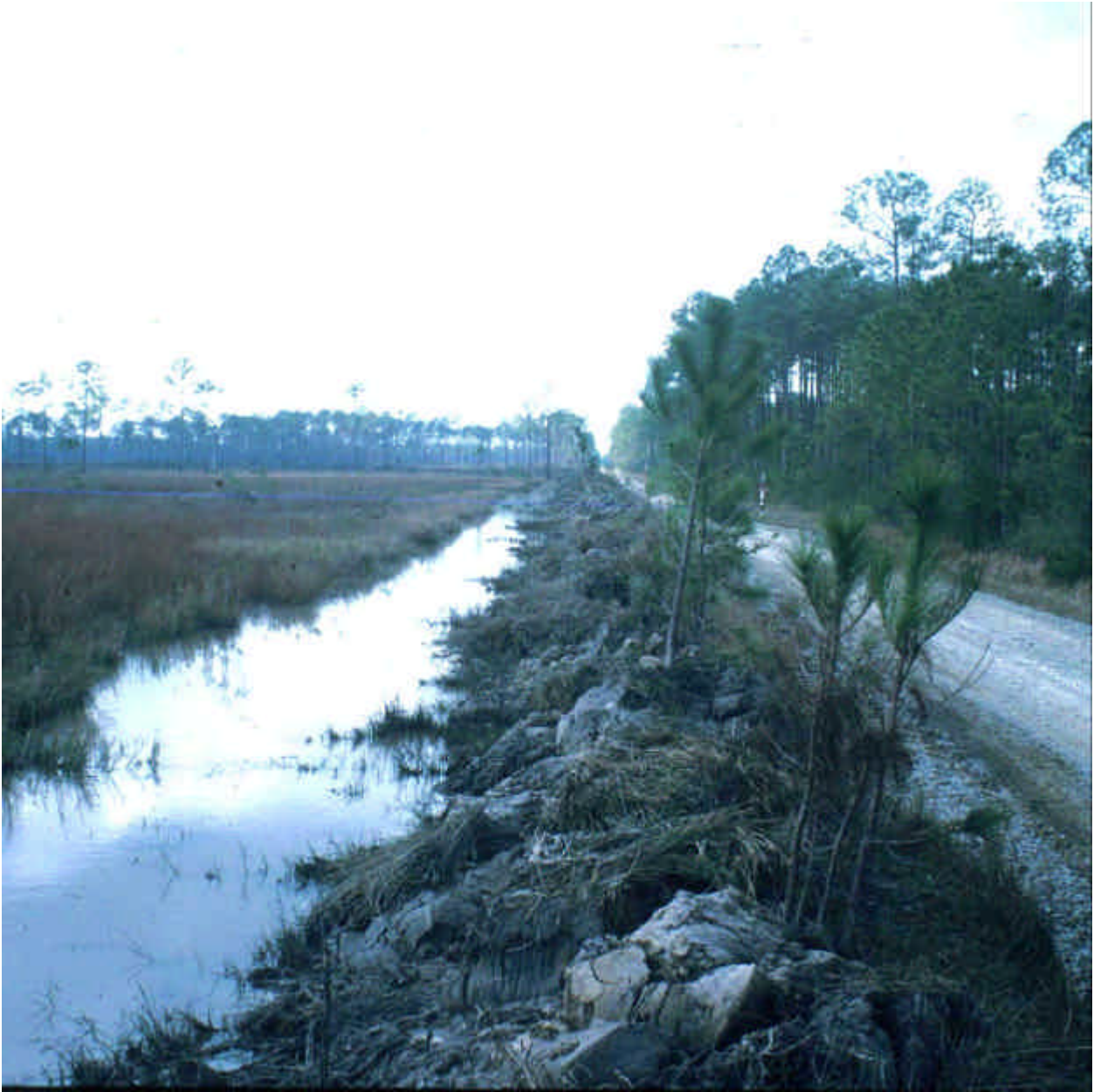
29. Road damming water in a Bunchgrass/Pine Savanna: left side is upgradient
