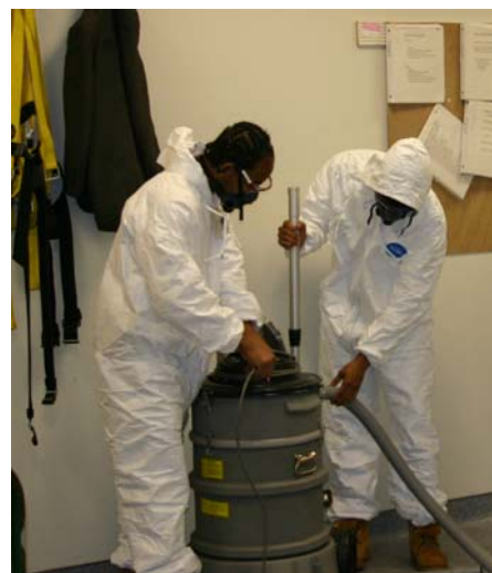
NJ/NY lead abatement exercise.
