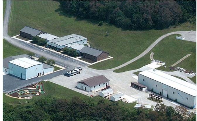
"Gold Standard" Laborers-AGC West Virginia Training Facility.
