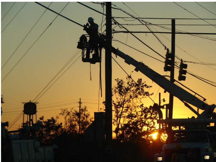
Restoring power after Katrina.
