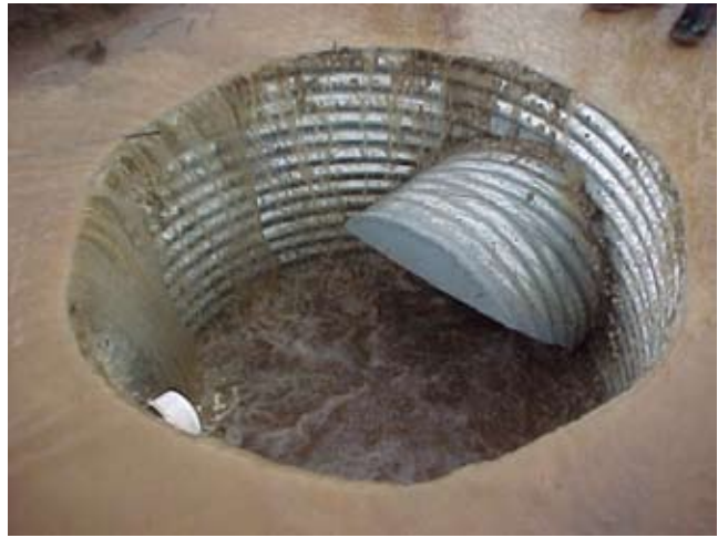
Figure 13–37 Riser with canopy barrel inlet
