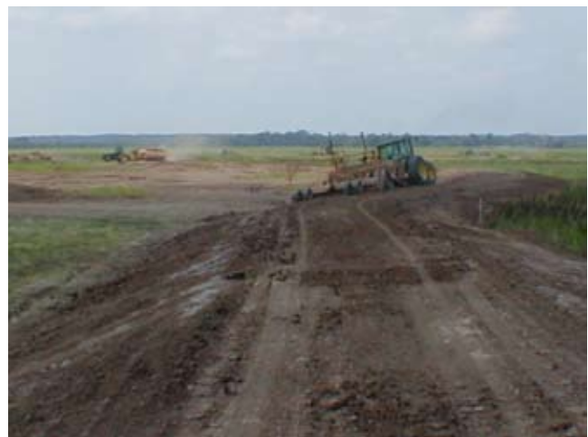
Figure 13–25 Dike for internal water control
