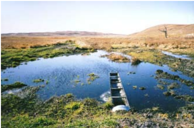
Figure 13–30 Cut pipe culvert
