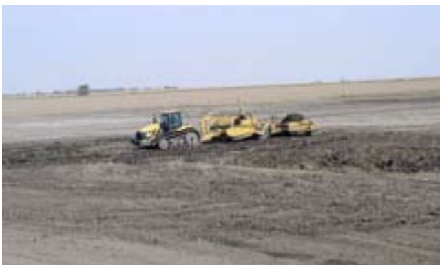
Figure 13–52 Wetland construction often requires low ground pressure equipment
