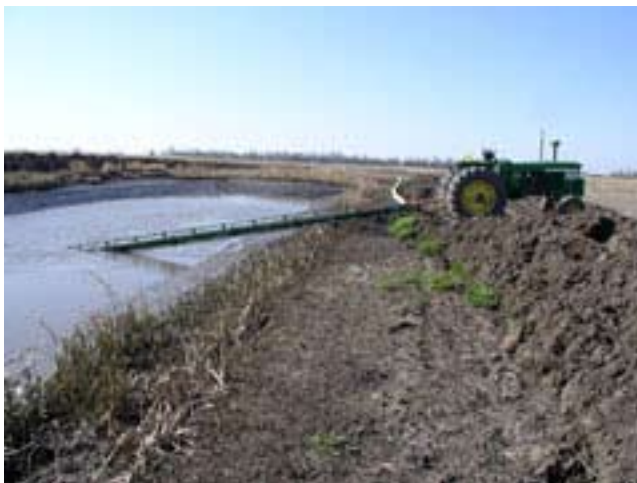
Figure 13–51 Dewatering a pit to be filled as part of restoration
