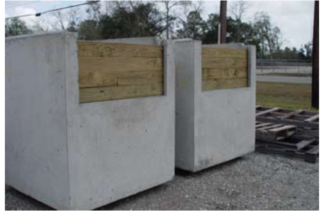
Figure 13-33 Pre-cast stoplog structures
