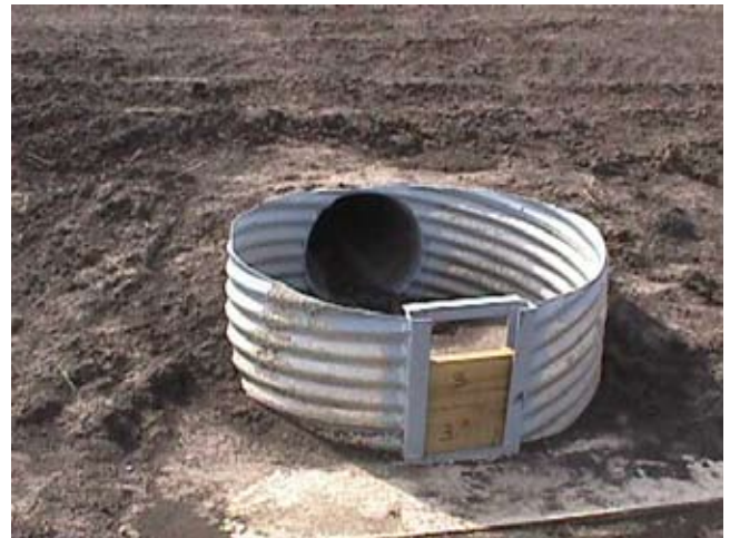
Figure 13-35 CMP riser with stoplogs
