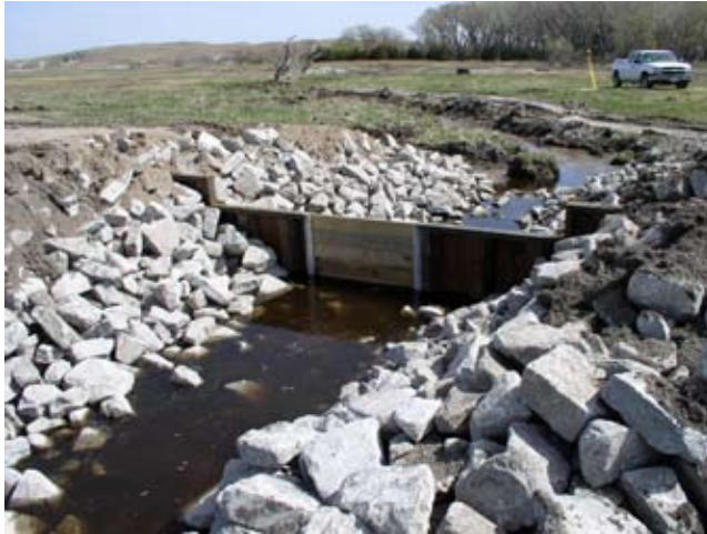
Figure 13-32 Sheet pile weir with stoplogs
