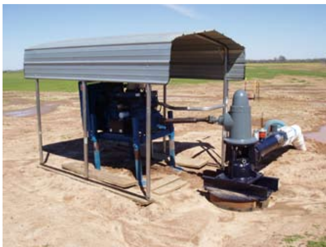
Figure 13–20 Hydrology enhancement with pumped ground water
