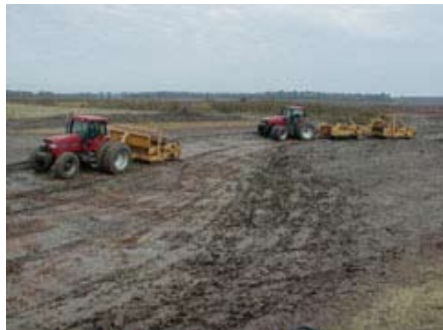
Figure 13–50 Construction in a riverine wetland project
