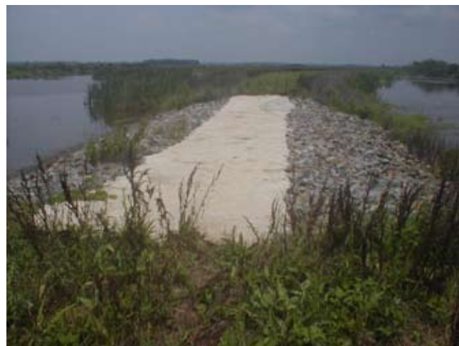
Figure 13-39 Armoring auxiliary spillway with concrete and riprap
