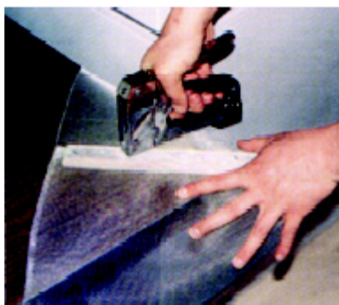
Figure 9A. Staple the longer edge of screening to the shorter piece of wood lath to form a cone.
