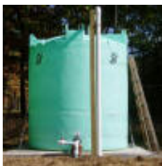
The Marion County Farm is utilizing an above ground tank for water storage.
