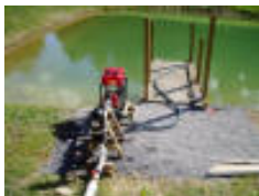
The Marion County Farm is using a pond to supply water for their irrigation needs. As you can see, he is utilizing a gasoline powered pump to siphon the water from the pond which then runs through a filter before being pumped up hill to an above ground storage tank.
