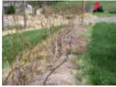
Monongalia County irrigation system for blueberry field. This picture was taken during the construction phase.
