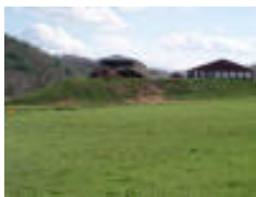
From left to right: terrace for additional windrow composting, litter sheds with mulch piles, and poultry houses.
