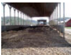
The front litter shed was built to NRCS specifications using EQIP funding. The shed contains composted turkeys.
